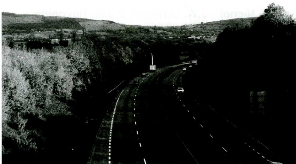
Fig. 1. A55 St Asaph Bypass cutting. View looking eastwards.
