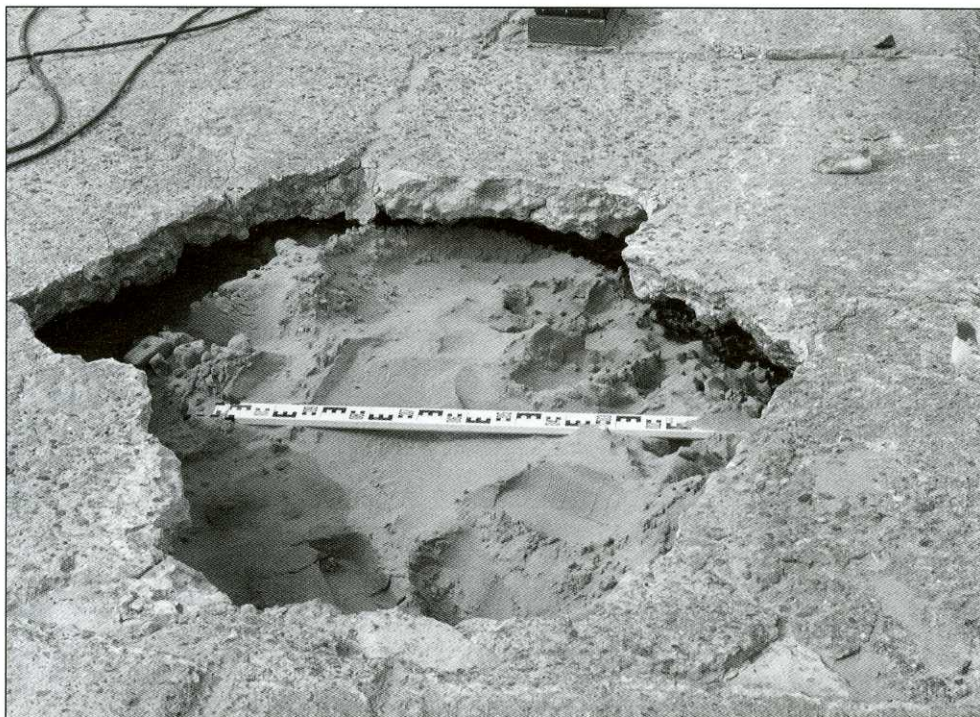
Fig. 3. Collapse feature (after infilling with sand for reasons of safety) on East Promenade, Rhyl, 17 April 1998. Photograph by Douglas Nichol
