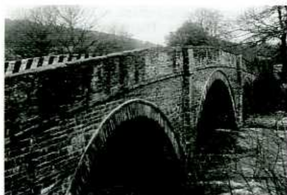
Fig. 3. View of Pont Melin Rŭg.
