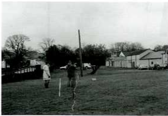
Fig. 6. Setting out Line 1. View looking westwards. Pont Melin Rûg on the left of the picture.
