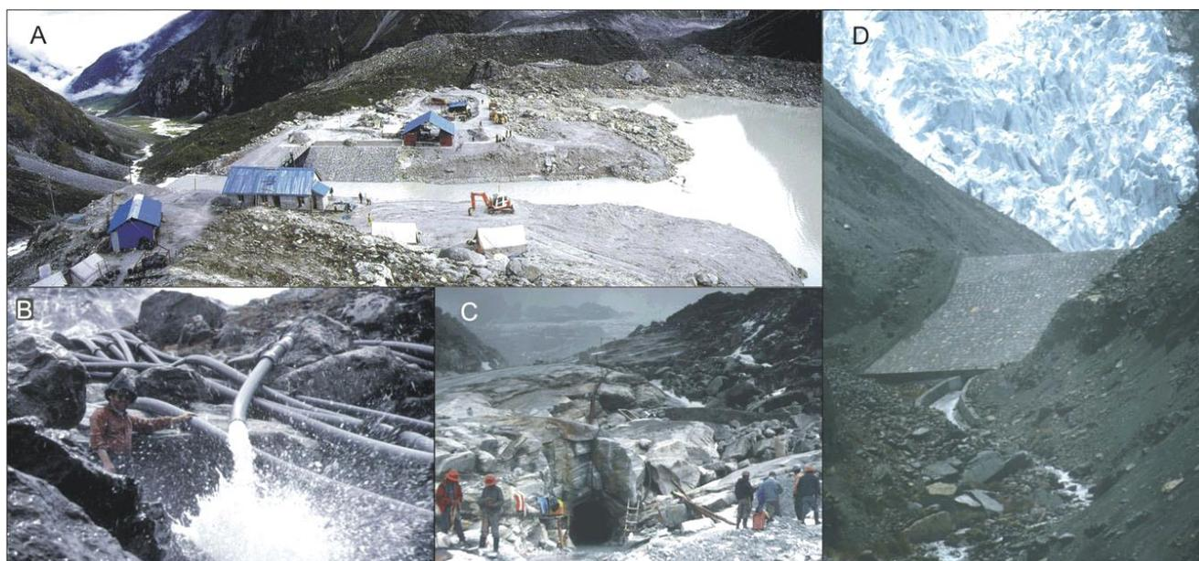
**Fig. 15:** Examples of glacial lake hazard remediation styles. A - channel with control gates, Tsho Rolpa, Nepal; B - Siphons, Tsho Rolpa, Nepal; C - tunnel through bedrock cored moraine dam, Lake 513, Peru; D - channel and reconstructed dam, Cuchillacocha, Peru (photo César Portocarrero).
