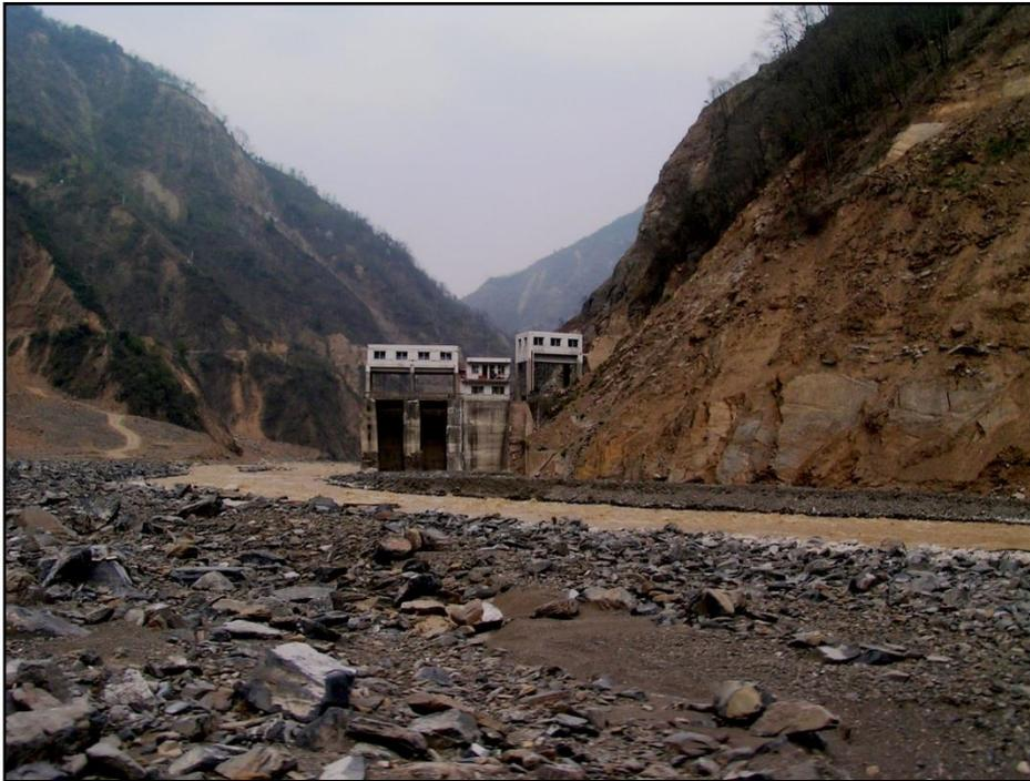
**Figure 1:** Remnants of the small hydropower structure downstream of the Tangjiashan landslide dam near Beichuan, Sechnan Province, China. The central sluice gates were swept away. (Photo courtesy of Dr Dave Petley).
