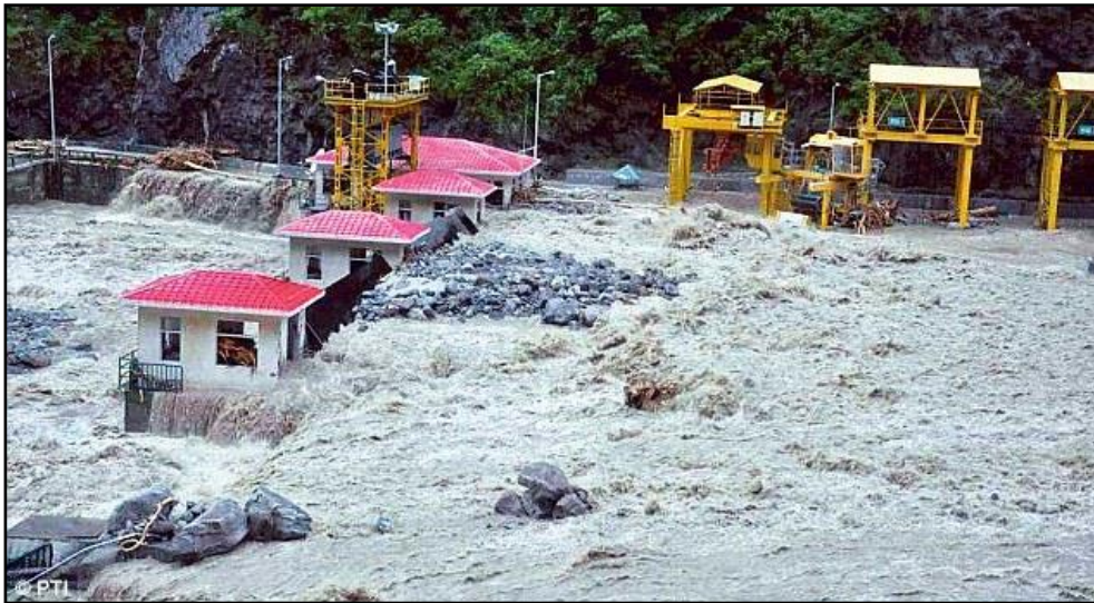
Figure 1: Vishnuprayag Hydropower Plant sluice gates being inundated and destroyed by the floods in Uttarakhand, northern India, in June 2013. (Image courtesy of www.thehindubusinessline.com ).
